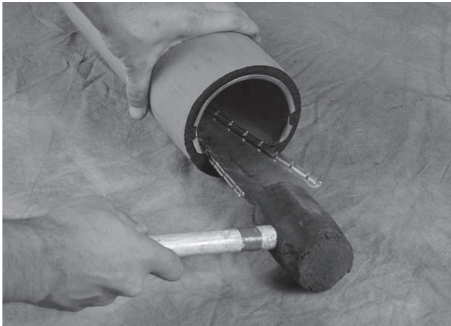
Figure 12 Install Split Ring Stiffener in PE Pipe
