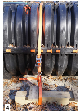
Position strap on beam.
