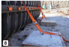
8 Connect strap to plate.
