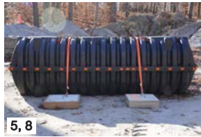
5, 8 Position straps on tank.
