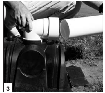
Connect inlet pipe.
