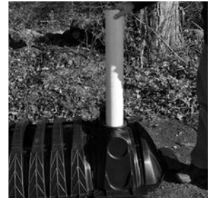
2. Pipe in endcap inspection port.
