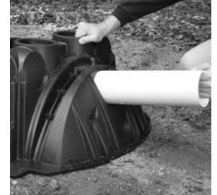
5. Insert inlet pipe.
