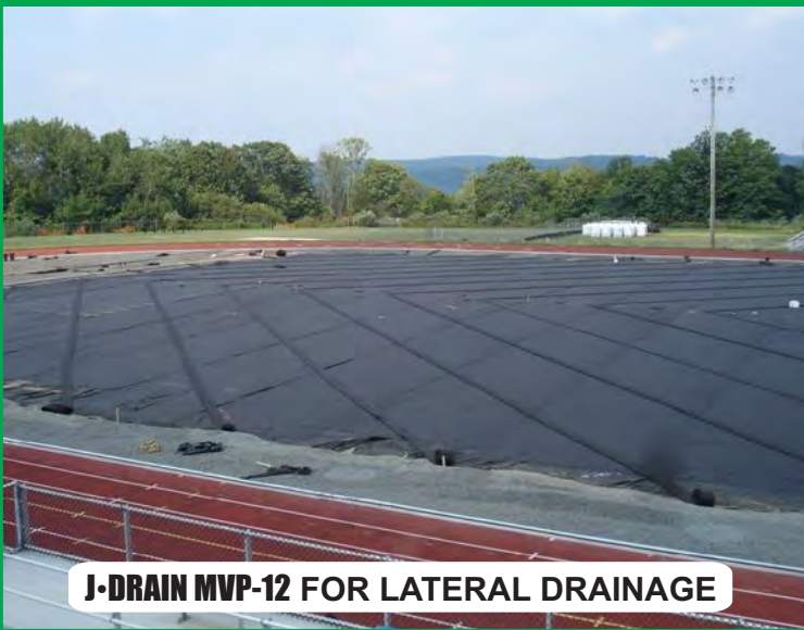
DRAINAGE LATERALS INTO SIDELINE TRENCH
