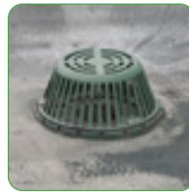
1. Remove sediment and debris around drain.
