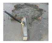
**1. Remove sediment** from the sides of the filter by sweeping away from Inlet Filter.
