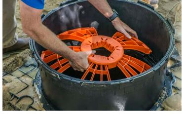
**1.** Install the Safety Star at the EZsnap narrow riser to riser connection closest to the ground surface. A minimum of a 6" (150 mm) riser is required to accommodate the Safety Star and to attach the lid properly.
