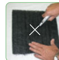
3. To ensure a snug fit, cut two slits on net side to make an X-shaped opening the size of the strainer.
