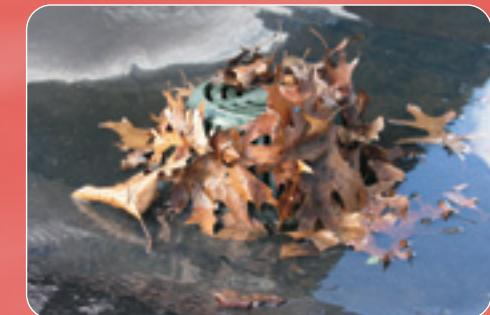
Easy to install roof drain filter keeps debris away from drain to allow water to drain.
