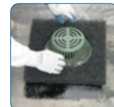
Apply adhesive to secure Filter to roof. Use Roofing Cement on asphalt membrane. Use water-based adhesive to secure to synthetic roof membrane.
