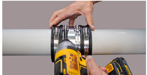
6. Center the coupling and tighten the bands.
