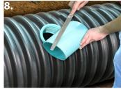
Bevel the leading edge of the pipe stub for easier insertion into the QwikSeal.
