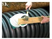
Install pipe fitting. Fitting should sit flush with the surface of the QwikSeal.
