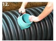
Install the band clamp at 60 in-lbs. torque.
