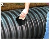
Using sand paper or a file, clean and remove any burrs from opening.
