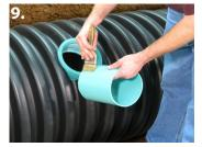
Lubricate the QwikSeal and pipe stub.
