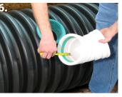
Measure the depth of the fitting to be attached pipe stub. See alternative method below.
