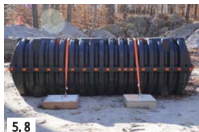
Position straps on tank.
