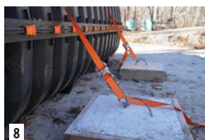
Connect strap to plate.
