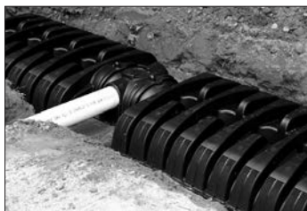
All-in-One 8 as mid-line connection.
