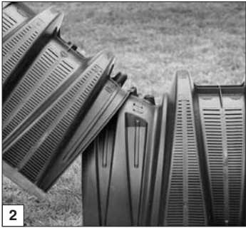
2 Connect the chambers.
