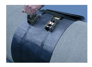
designed to prevent inflow/infiltration and exfiltration at the joint. In addition, MacWrap CR is proven to maintain the joint integrity, even given less than perfect bedding conditions.
