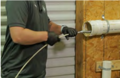
STEP 1 Inspection & Preparation
