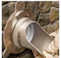
Solvent weld nozzle onto pipe and into escutcheon. Dura G-O-N requires the mounting notch in the escutcheon and the nozzle be aligned for proper contact.
