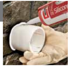
Caulk wall opening.
